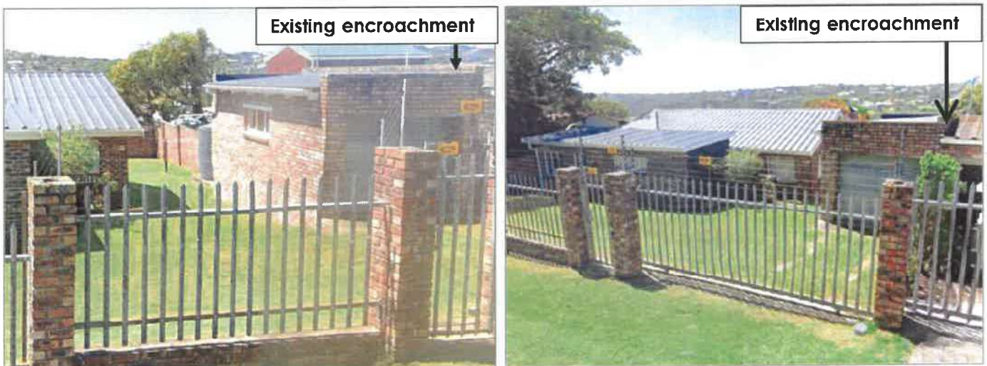
Existing garage encroaching the 1,5m south-eastern lateral building line:
